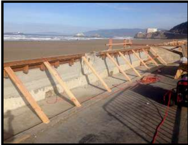
Ocean Beach Seawall Repairs, SF
