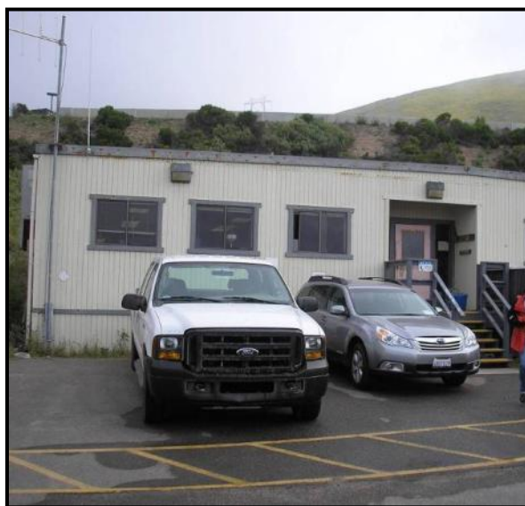
Figure 2-6. Existing Onshore Data Collection Building
