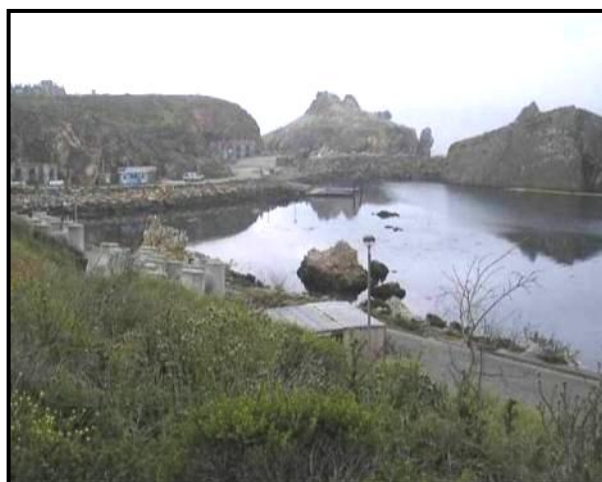
Figure 2-9. Existing Boat Dock within DCPP Intake Embayment
