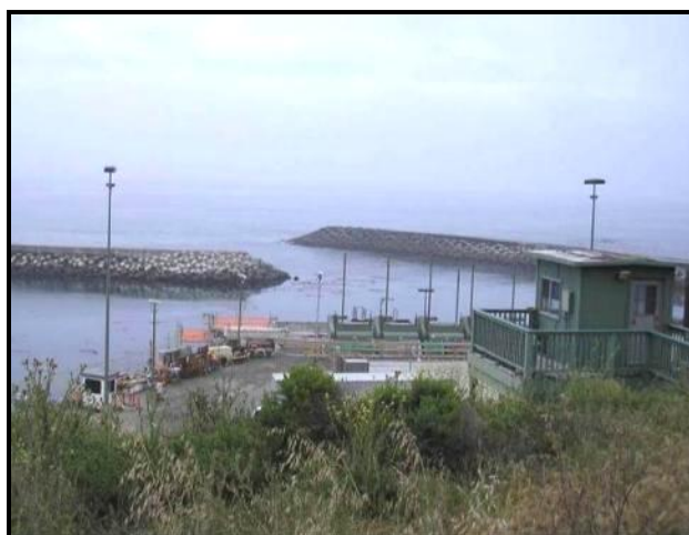
Figure 2-8. Intake Embayment Entrance
